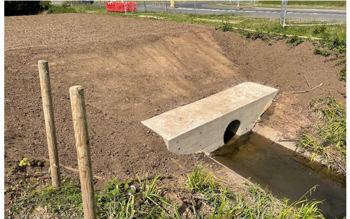
Plate 4-22 Example Culvert Installation for Water Crossings (Source: Dogger Bank C)
