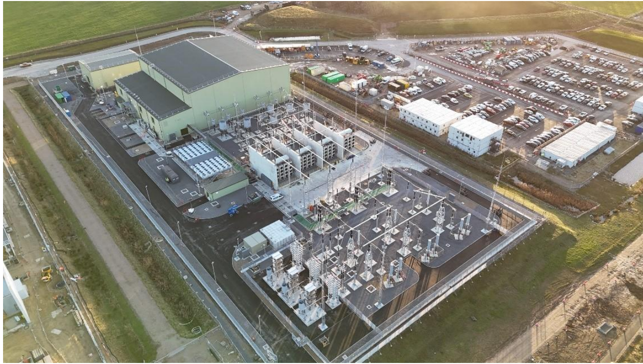
Plate 4-23 Example Onshore Converter Station (in construction) (Source: Dogger Bank C)
