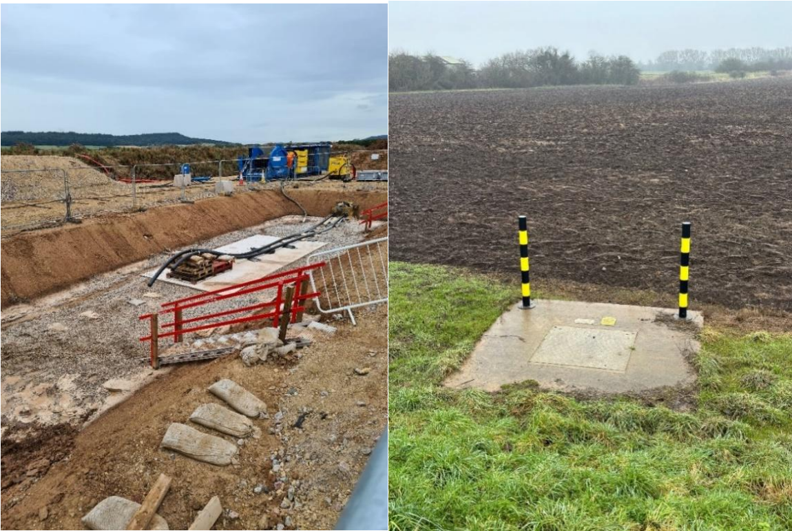
Plate 4-12 Example TJB during Construction (Left) (Source: Dogger Bank C) and Example Underground Link Box during Operation (Right, Note: Only manhole cover to the underground link box, and demarcation posts (where required) will be visible at ground level) (Source: Dogger Bank A & B)
