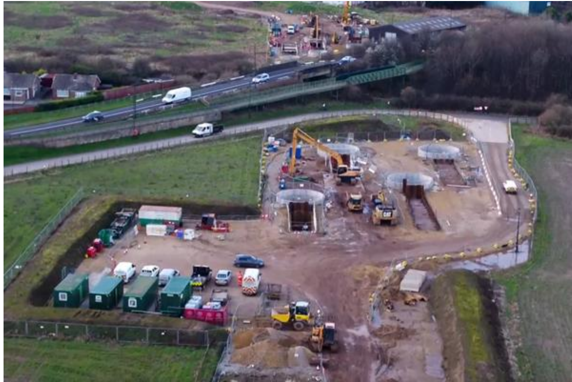
Plate 4-18 Example Trenchless Installation Compound for Onshore Export Cable Works (Note: Compound dependent on the selected trenchless installation technique at each crossing) (Source: Dogger Bank C)
