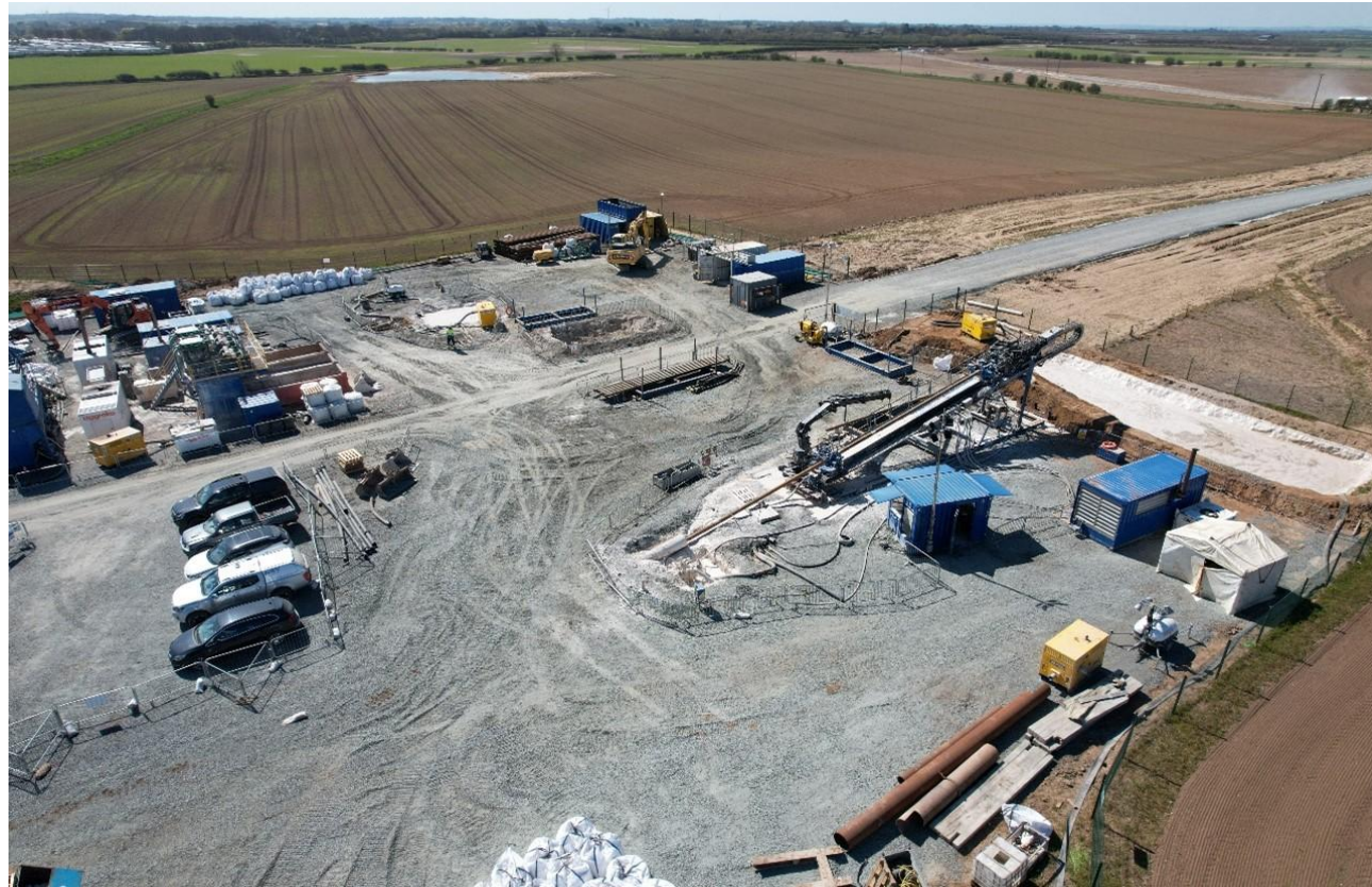
Plate 4-13 Example of a Landfall Construction Compound (Note: Compound will be dependent on the selected trenchless installation technique at landfall) (Source: Dogger Bank A & B)
