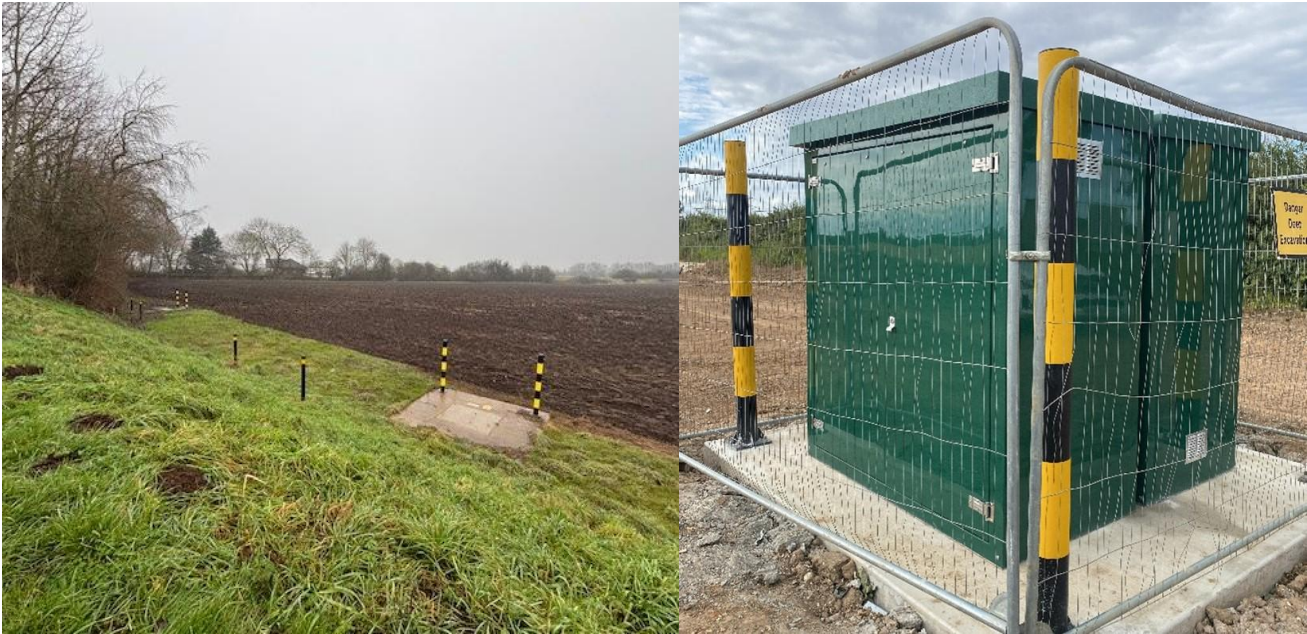
Plate 4-15 Example of an Underground Link Box (Left) ((Source: Dogger Bank A & B) and an Above-Ground Link Box (Right) (Note: This includes temporary fencing during construction) (Source: Dogger Bank B)
